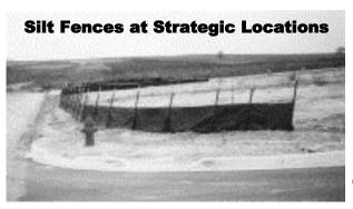
Properly located and installed silt fences can greatly reduce the amount of sediment that leaves a construction site.
